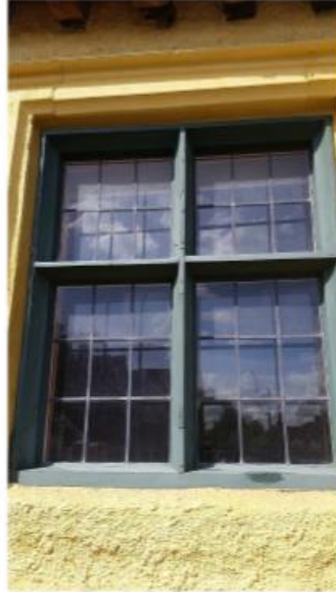
Detail view of one of the windows in the north elevation showing the traditional joinery framing to the glazing
